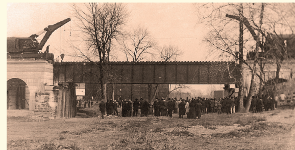
Ephrata Township: Now renovated for trail use, the steel bridge crossing the Cocalico Creek is shown here during its construction in 1909, replacing an earlier wooden structure and allowing the Reading & Columbia line to use heavier locomotives.
